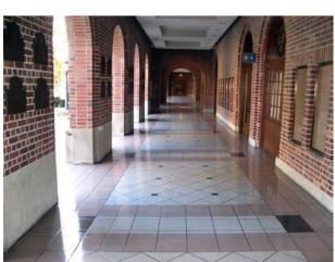
removing and replacing the tile, placing mats over the tile or utilizing the polymeric properties of SlipShield 1000. SlipShield 1000 was selected and applied to the ceramic tile portico area and the ceramic tile steps in order to preserve the aesthetic quality of the ceramic tile floor system.
